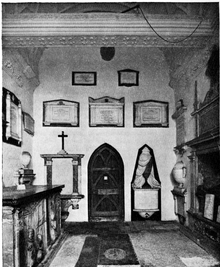
Lumley Chapel of St. Dunstan's, Cheam, Surrey: the West wall. (Before restoration)
